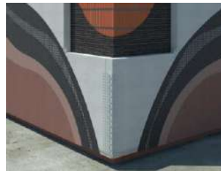
U = 0,41 \text{ W/m}^2\text{K} SATE EPS de 8,00cm
